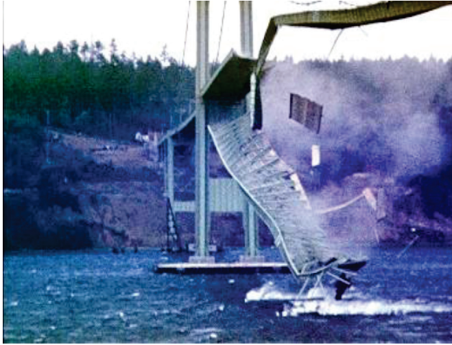
Fig.3-16; Vibrations breaking the bridge
