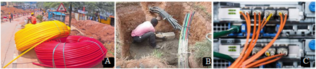
Fig.5. 1: The installation and use of optical fiber in Rwanda
