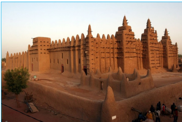
Fig. 17.3: The Great Mosque of Djenné in Mali
