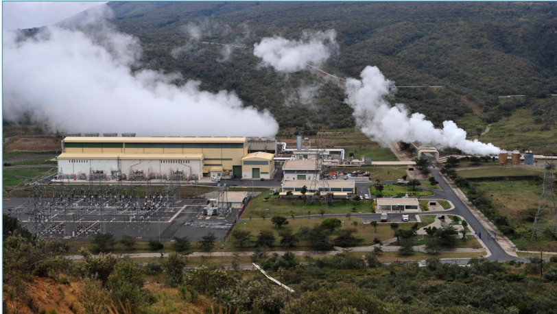
Fig. 14.3: Olkaria geothermal station in Kenya
