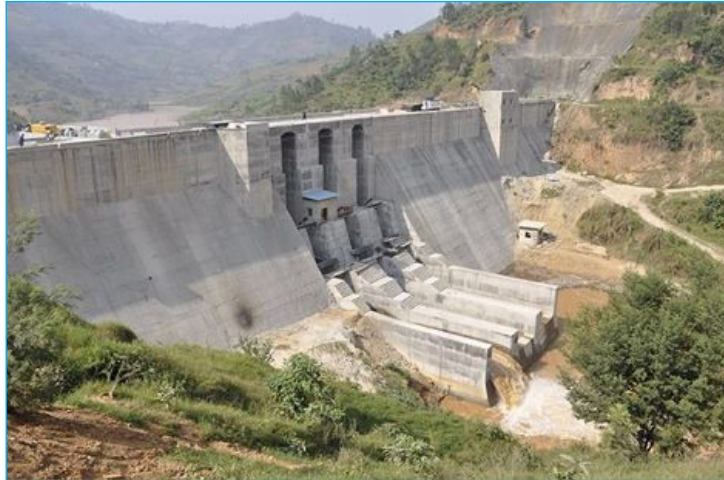
Fig. 6.5: H.E.P station on River Nyabarongo
