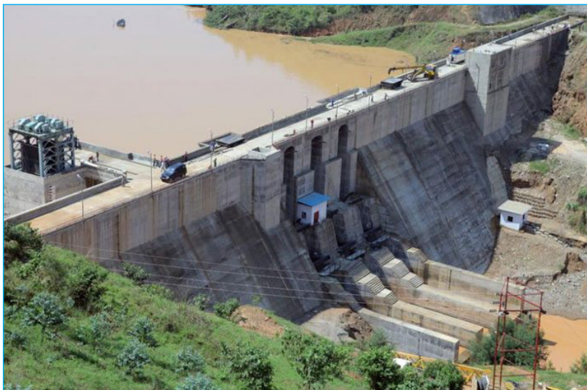
Fig. 14.2: A hydro-electric power station on River Nyabarongo
