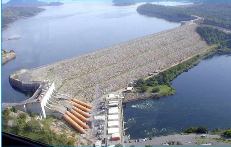
Fig. 14.7: Akosombo Dam on River Volta
