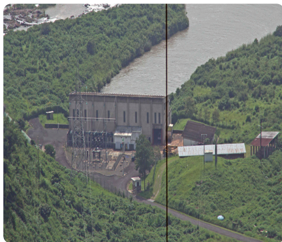
Fig 15.8 Hydroelectric power project on Rusizi River
