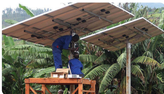
Fig 15.3 Technicians installing solar panels
