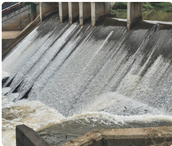
Fig 15.7 Mukungwa hydroelectric power generation
