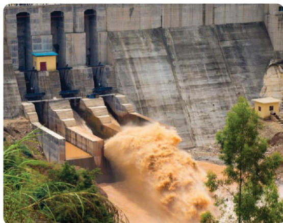
Fig 15.2 Nyabarongo hydropower plant in Muhanga district
