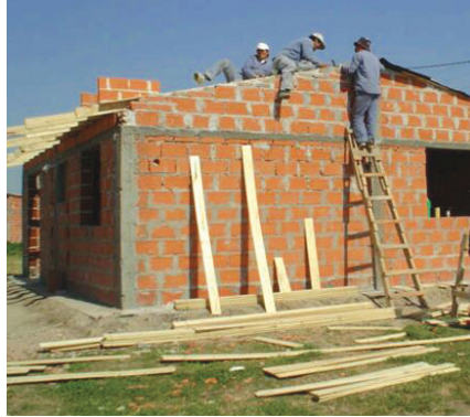
A house that is being built with bricks, cement and sand
