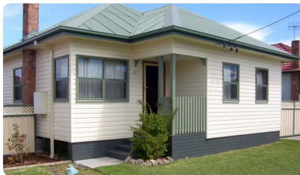
A house built with boards and iron sheets
