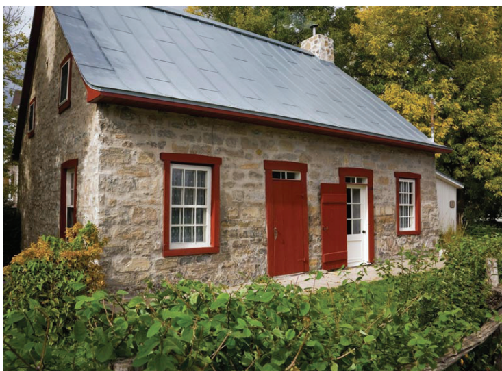
A house built with stones and iron sheets
