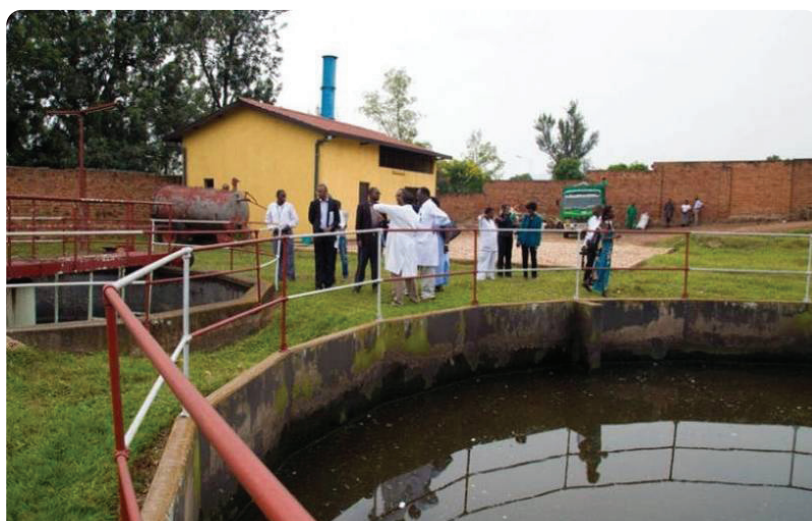
Fig 5.6: Sewage treatment plant in kigali city
