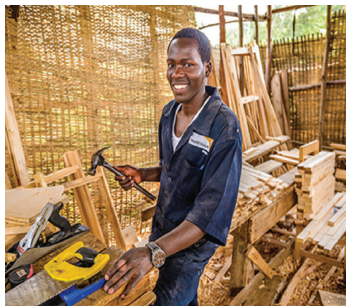
Carpenter at work
