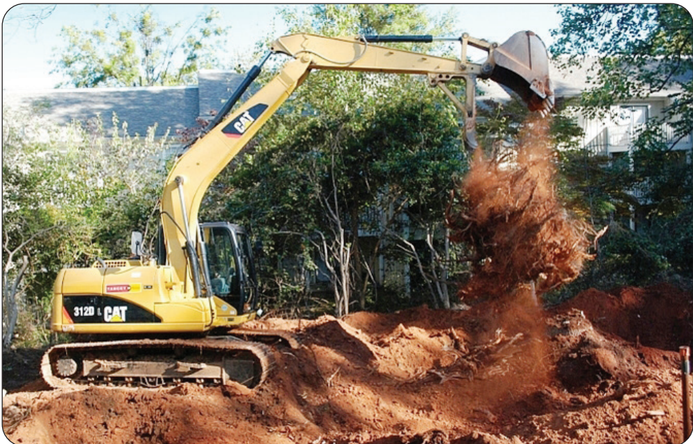
Fig. 1.64: Excavating the site for gabion placement
