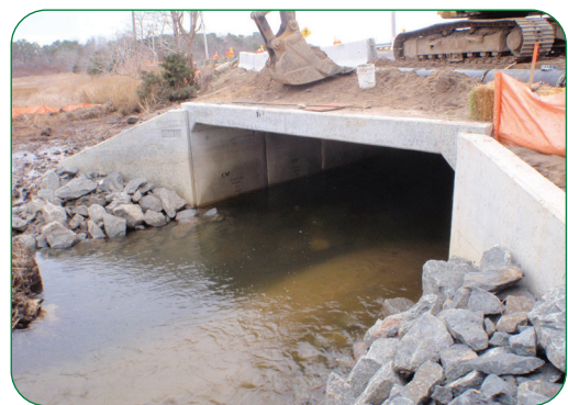
Fig. 1.16:(b) Culvert constructed to lead water
