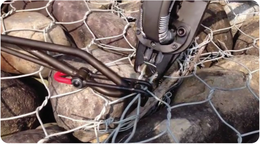
Fig. 1.67: Closing gabion boxes
