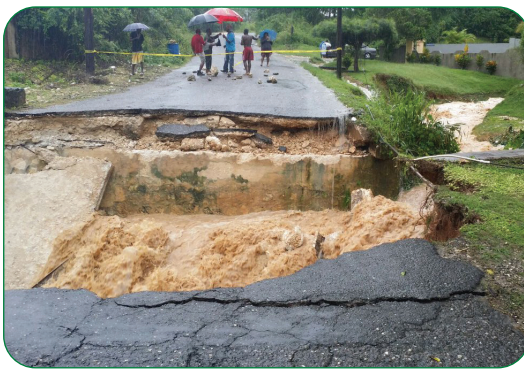
Fig. 1.16:(a) Road interfering with drainage
