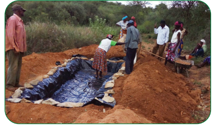
Fig. 4.13: Pit lined with polythene sheet
