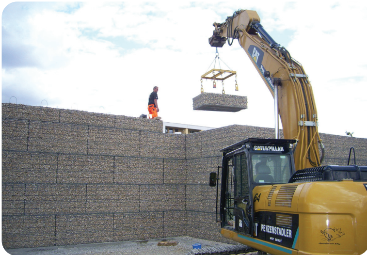
Fig. 1.68: Stacking gabion boxes together
