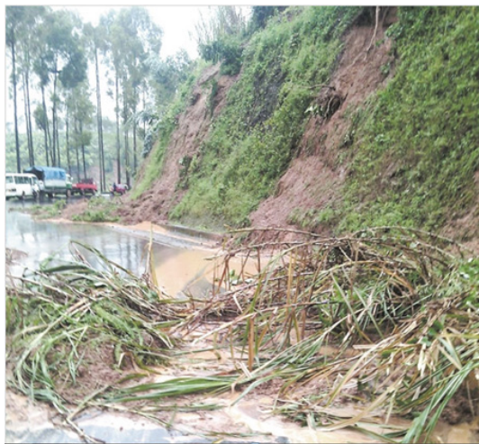
Floods and landslides
