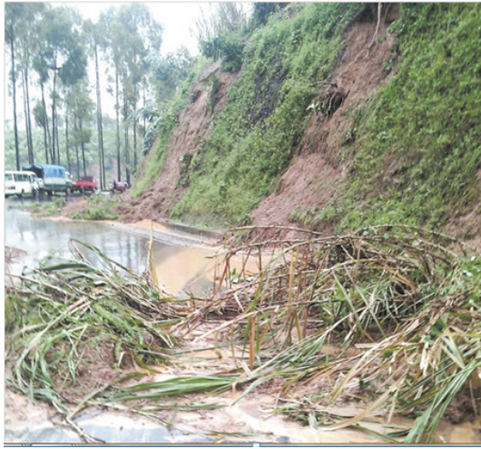
Flooding and landslides
