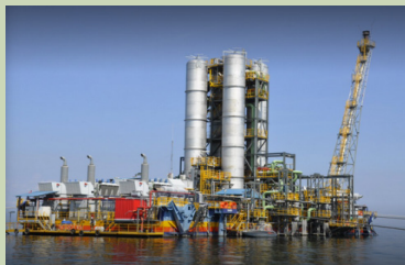
Picture 2.1: Kivu watt power station
