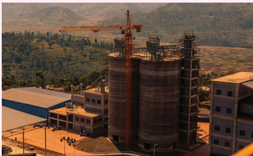
CIMERWA cement factory, Muganza sector, Rusizi district
