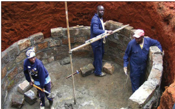
Figure 6.8: Construction works of the digester chamber for a fixed dome bio-gas plant. Biogas will play a key role in reducing pressure on the country's forests
