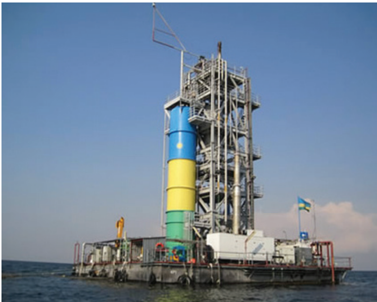
Figure 6.2: A methane gas extraction plant on Lake Kivu
