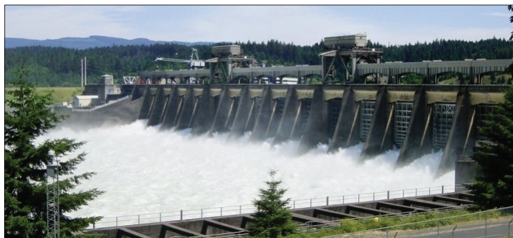
Figure 6.14: Hydroelectric power station
