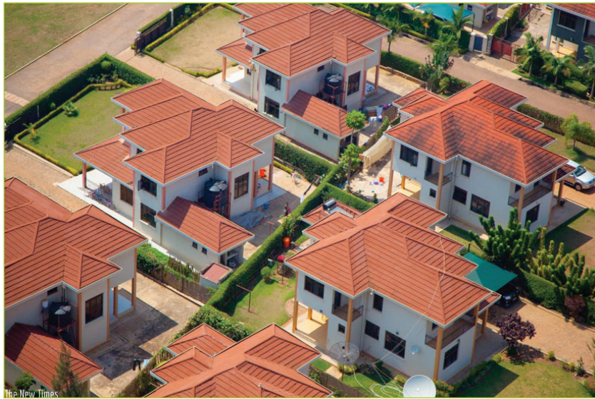
Fig 12.7 An Aerial view of housing units of urban settlements in Kibagabaga, Gasabo District.
