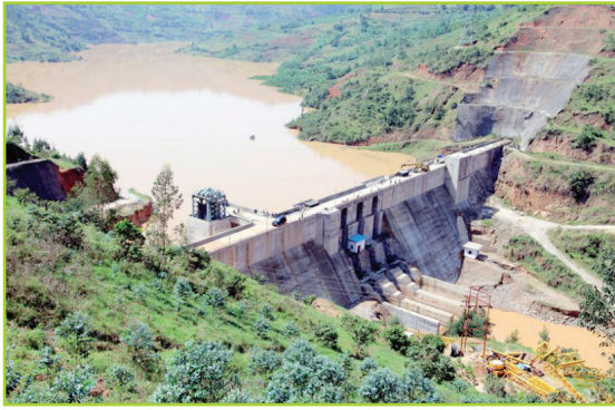
Fig 10.4 Dam on Nyabarongo River.
